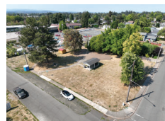
Corner View at I St. and 4th St.
