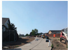
Concrete Circulation Path/Park Under Construction
