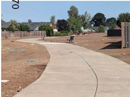
Concrete Circulation Path and Benches
