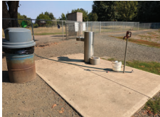
Trash, Water, and Storage Structure on Site
