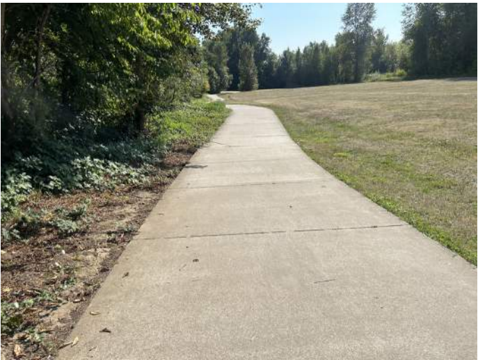
Willamette River Trail Concrete Path Connection
