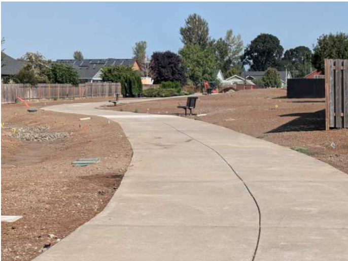
Concrete Circulation Path and Benches
