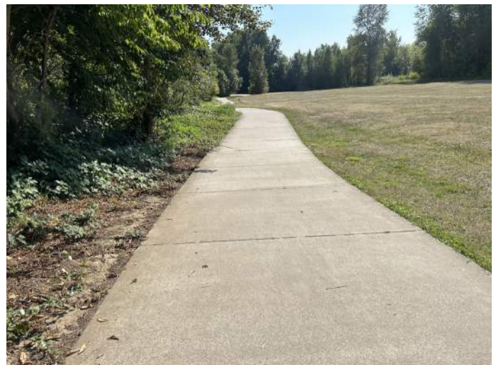
Willamette River Trail Concrete Path Connection
