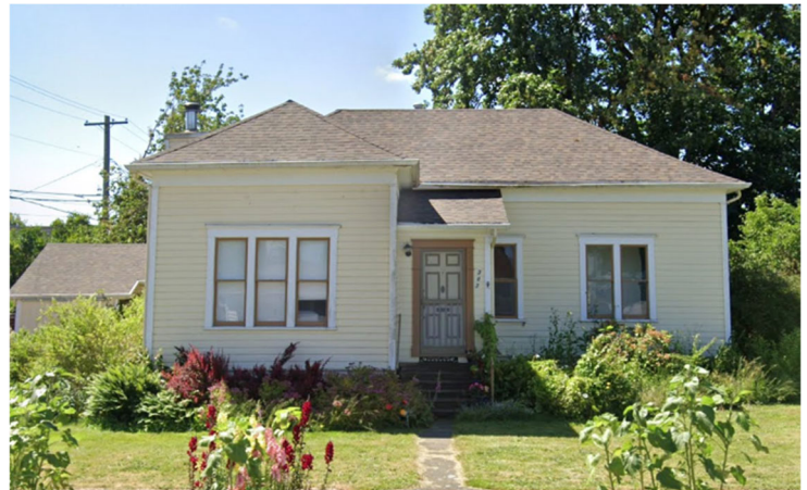
FIGURE 2: FRONT PHOTO OF BUILDING
