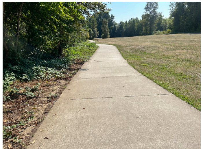
Willamette River Trail Concrete Path Connection
