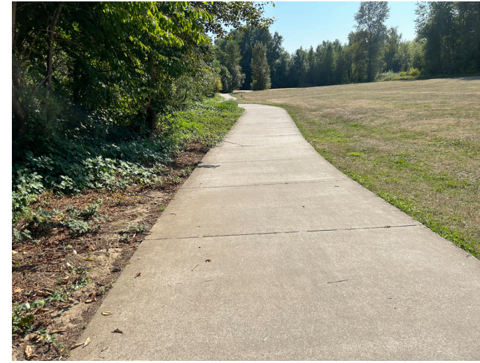
Willamette River Trail Concrete Path Connection
