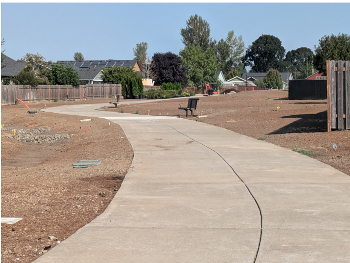
Concrete Circulation Path and Benches
