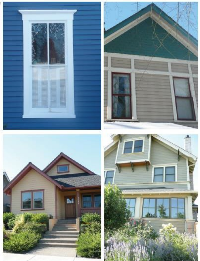
Trim. [1] All street-facing windows and doors shall have side trim and head casings [2] Trim shall be at a minimum 3½ inches wide and project no less than ½ an inch from the wall.
