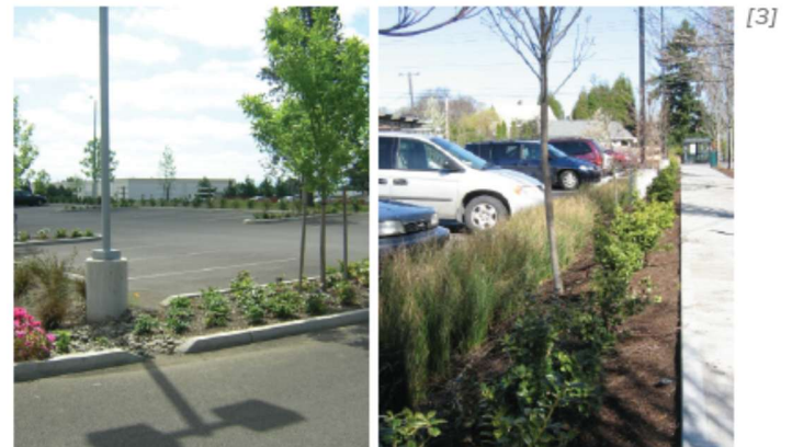
Off-Street Parking Lot Landscaping. Parking lot appearance and functionality can be improved by [1] a minimum perimeter setback of 6 feet with ground cover, shade trees, and shrubs that are a minimum of 3 feet high [2] internal landscaping strips that are a minimum of 8 feet wide [3] and stormwater detention and retention landscaping that reduces run-off while also providing a buffer between parking and pedestrians.
