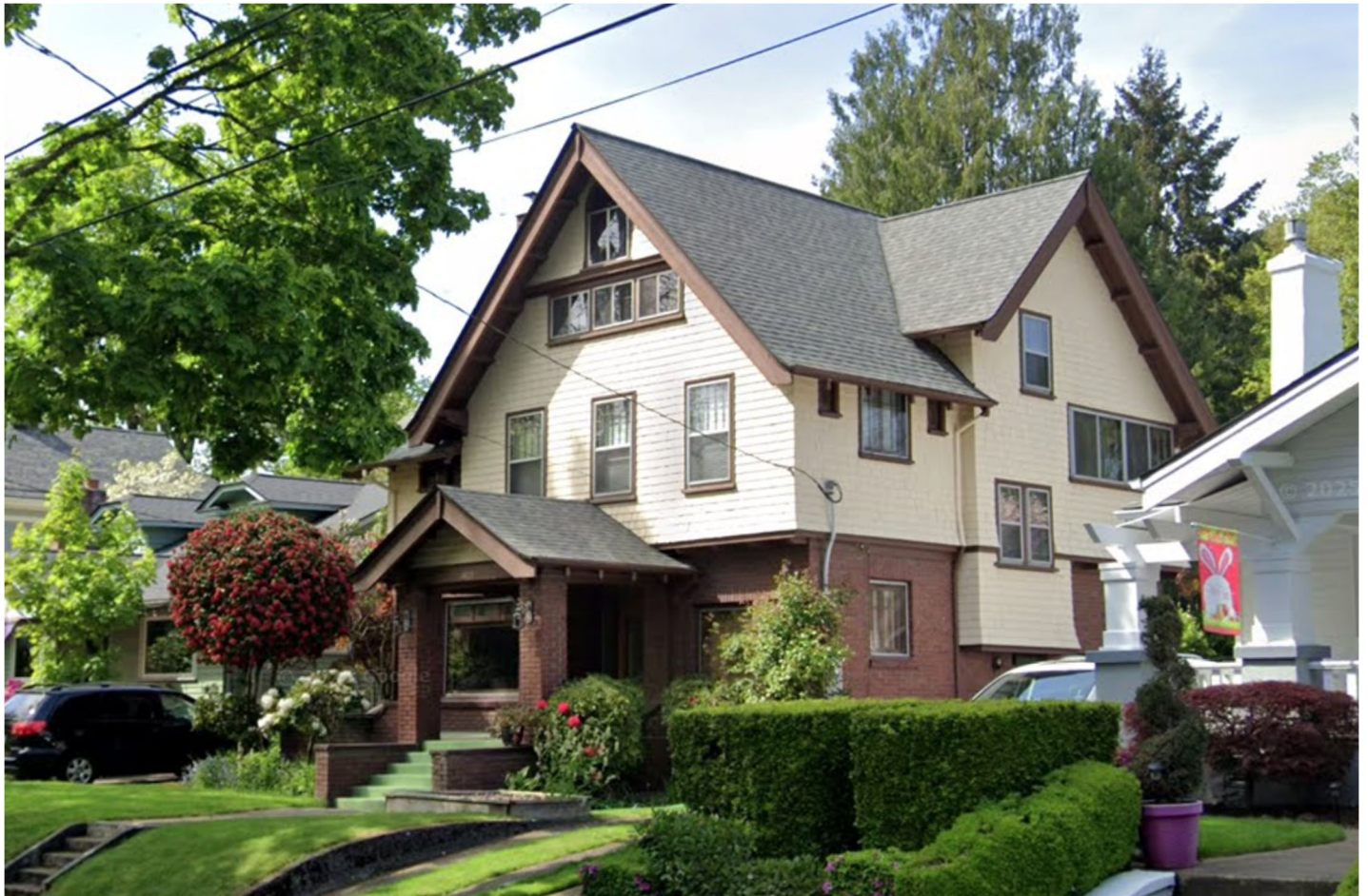
Home height to gable ~ 32-33 feet (4025 NE Couch)
