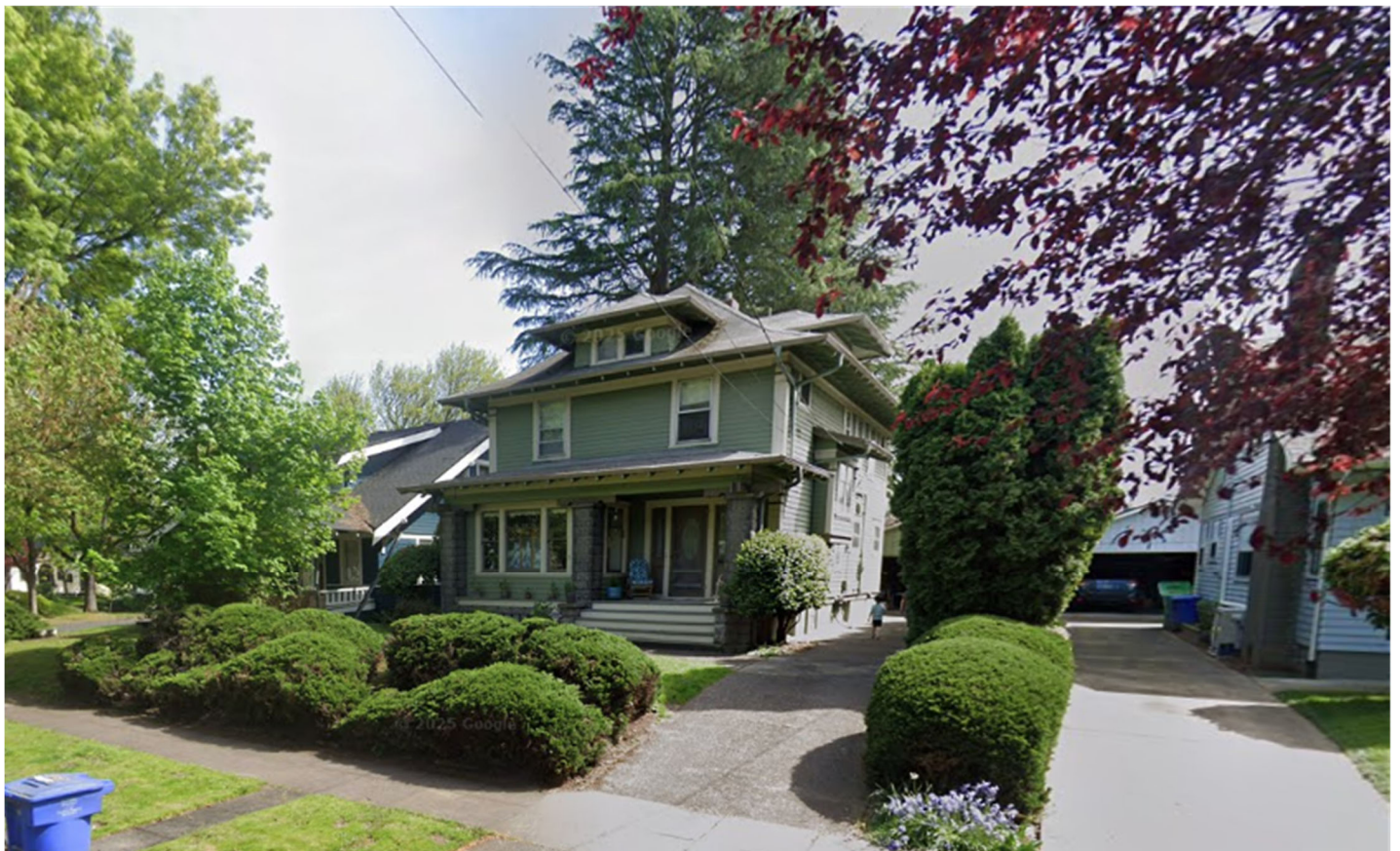
Home height to gable ~ 30 feet (4044 NE Couch)
